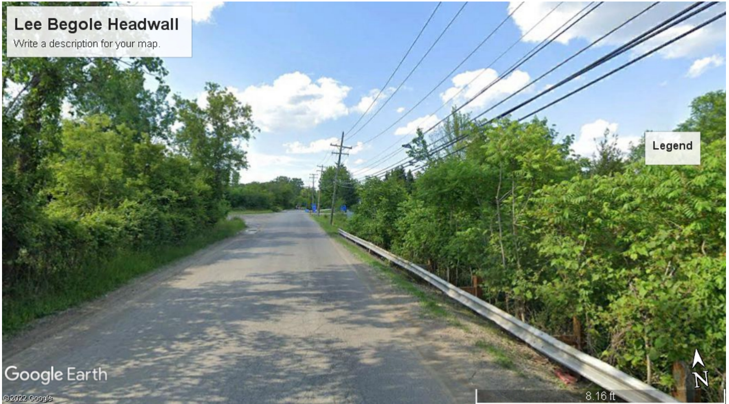
Before – Looking north on Lee BeGole Drive. Headwall on right in the vegetation.
