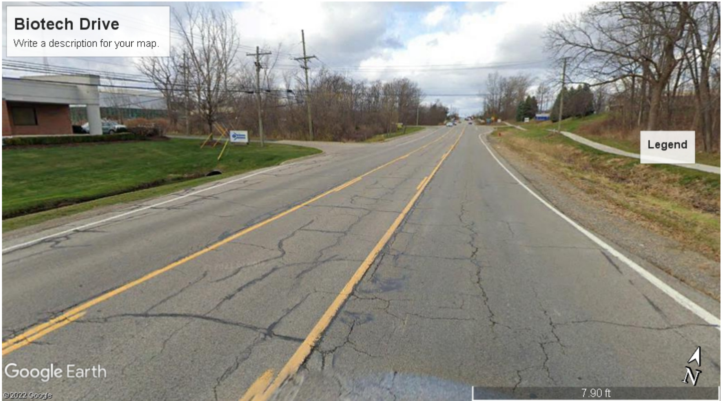
Before – Looking north on Meadowbrook Road, along the west side.
