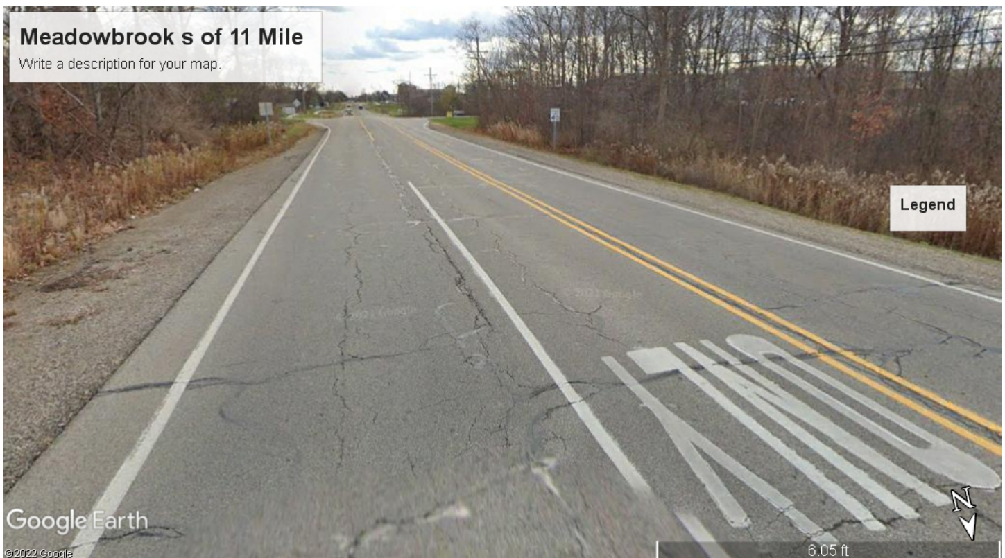
Before – Looking south on Meadowbrook Road, along the west side.
