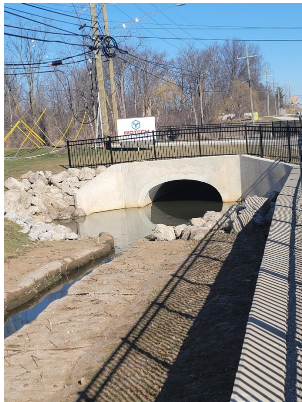
After – Completion of the culvert at Biotech and final Bishop Creek stabilization.
