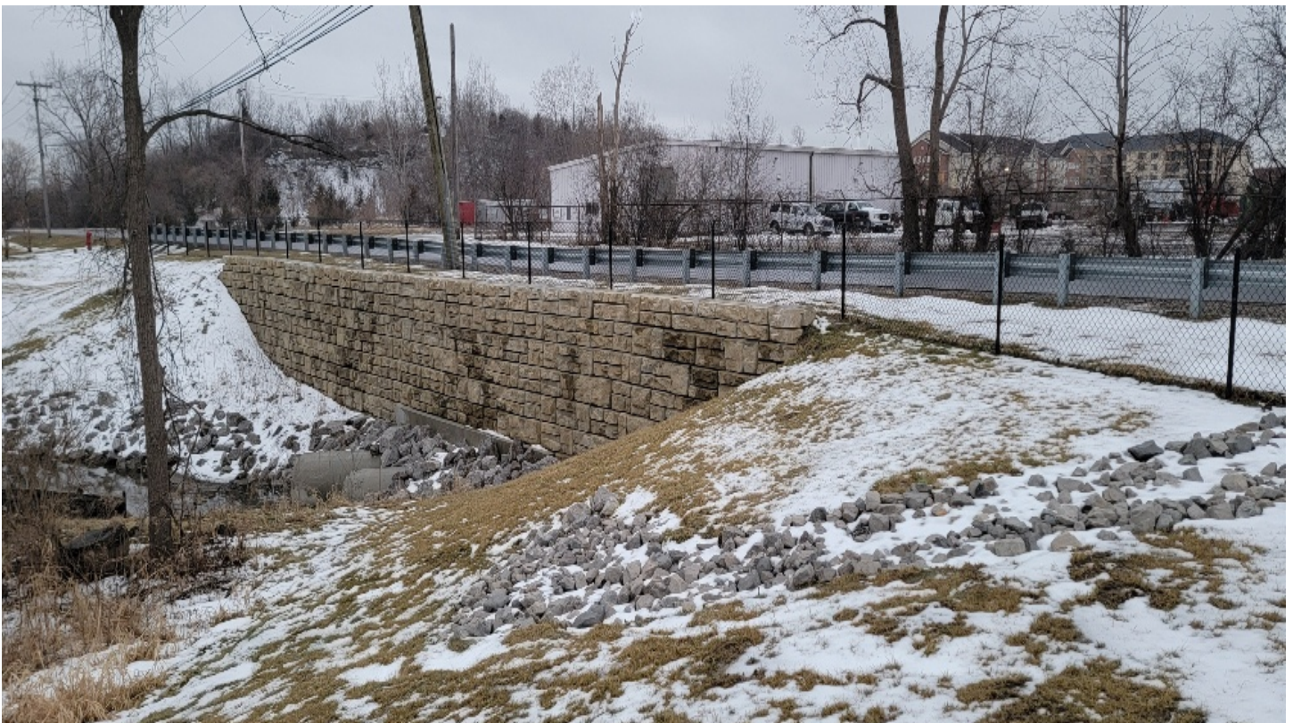
After – Looking at east-face of wall from DPW yard.
