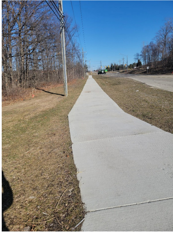
After – Completed segment of Meadowbrook Road sidewalk, south of 11 Mile Road.
