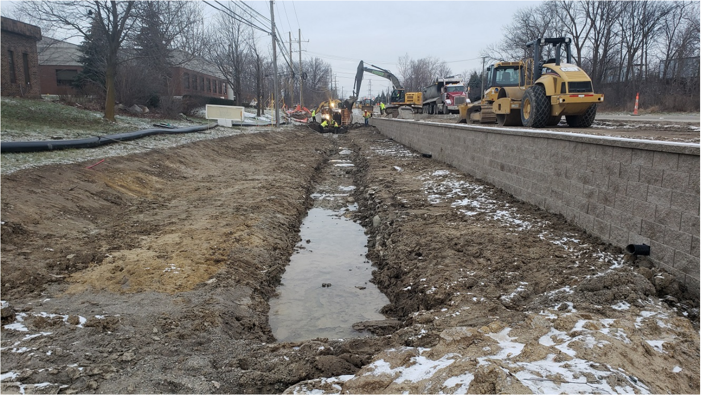
During – Completion of the retaining wall and reshaping of the Bishop Creek ditch.
