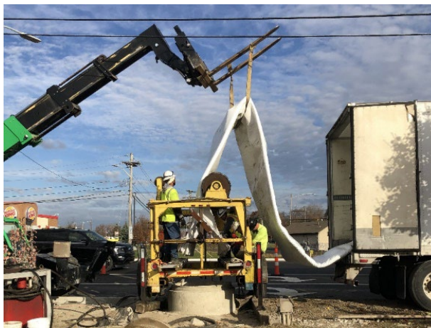
Figure 17: CIPP Felt Liner Inversion during Elizabeth Lake Road Sinkhole Sewer Rehabilitation
