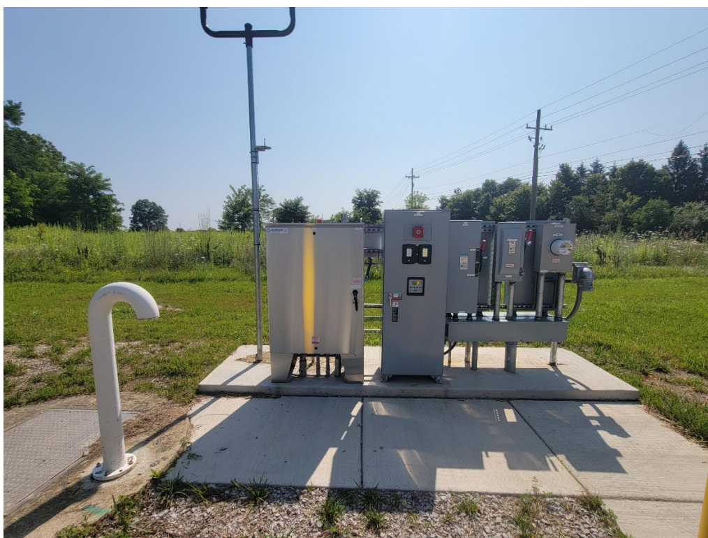
After – Placement of Pump Station equipment
