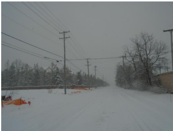
Trans X Road – Looking South
