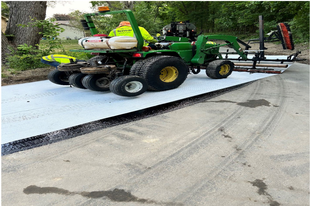
(After) Paramount Street at Linhart – Placement of Interlayer fabric before final asphalt wearing course
