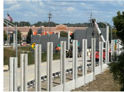
NB I-75 exit ramp to 12 Mile Road Noise wall construction
