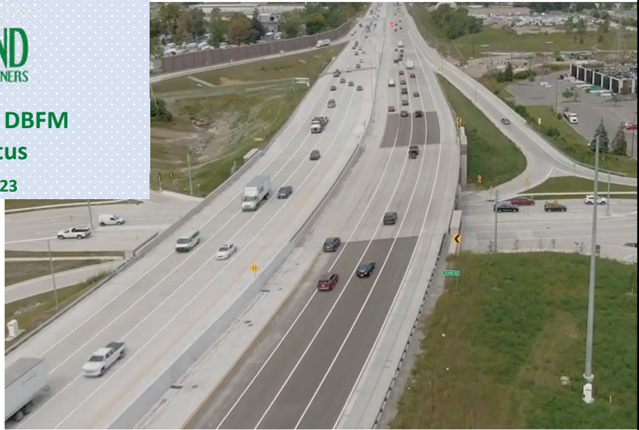
I-75/12 Mile Road Interchange looking north
