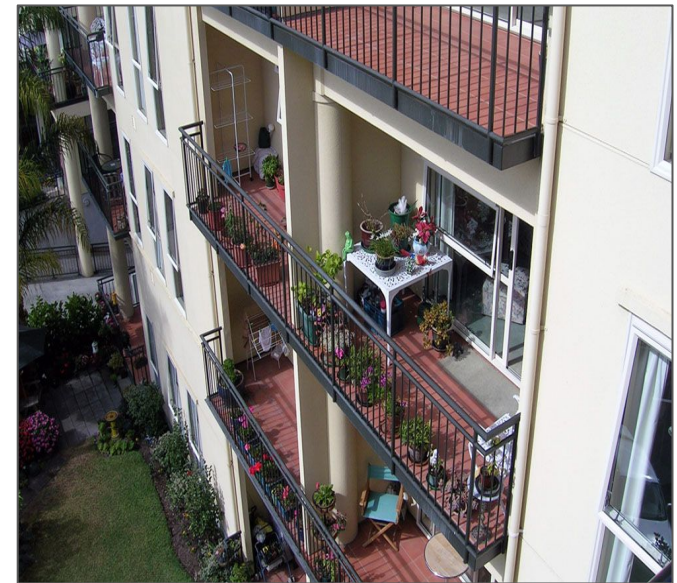
Dedicated outdoor space for every unit
