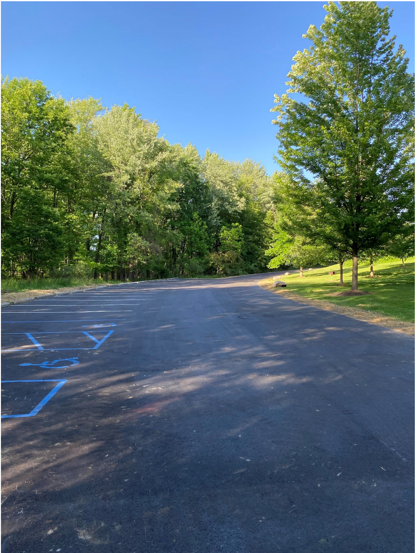
After – New north end of parking lot
