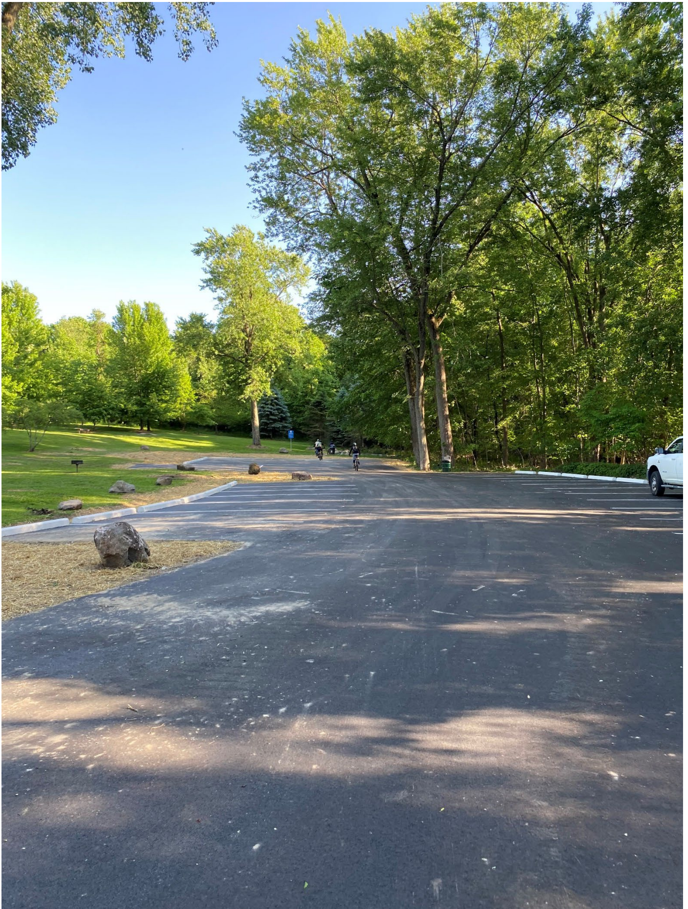
After – New south end of parking lot
