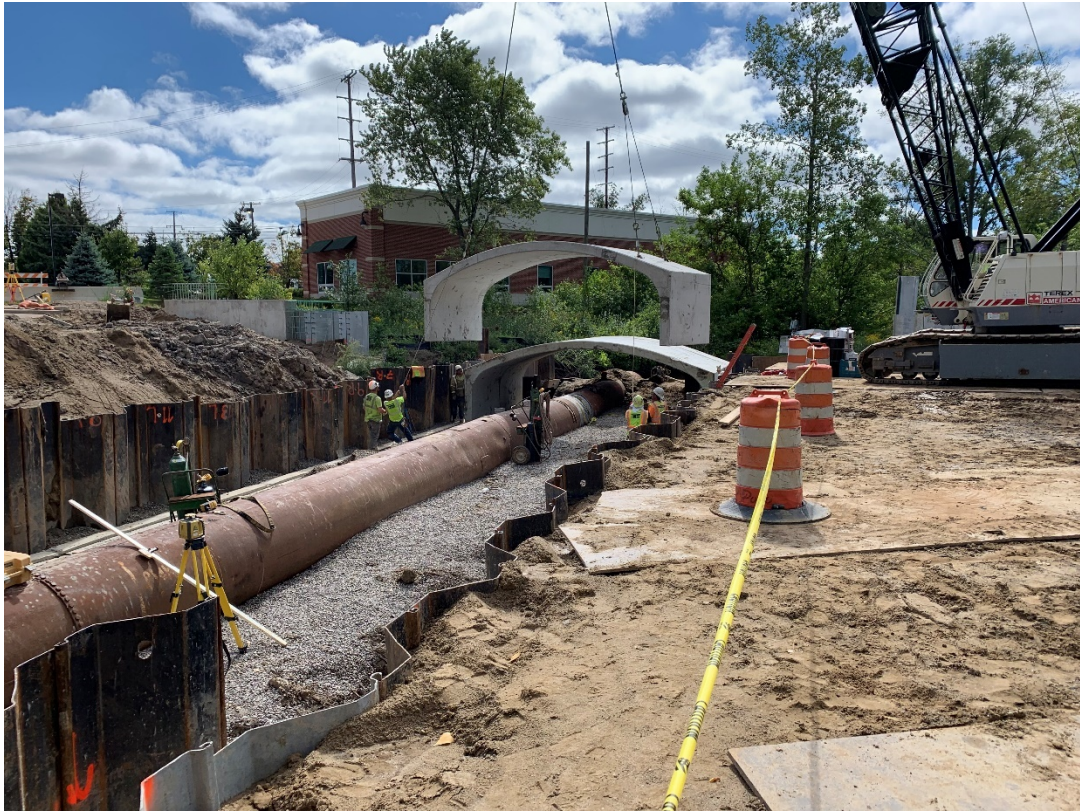
Installing the new modified box culvert over top the Middle Rouge River by-pass.
