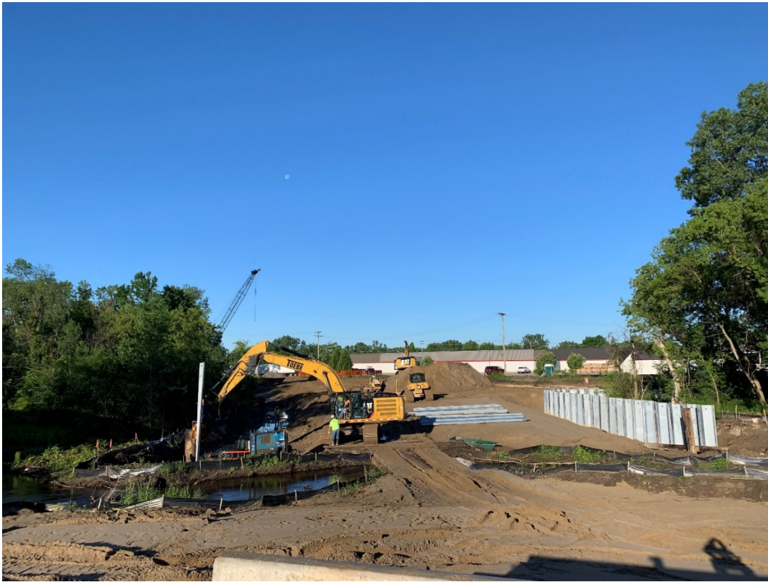
Installing sheeting and forms for the walls on each side of the Middle Rouge River.
