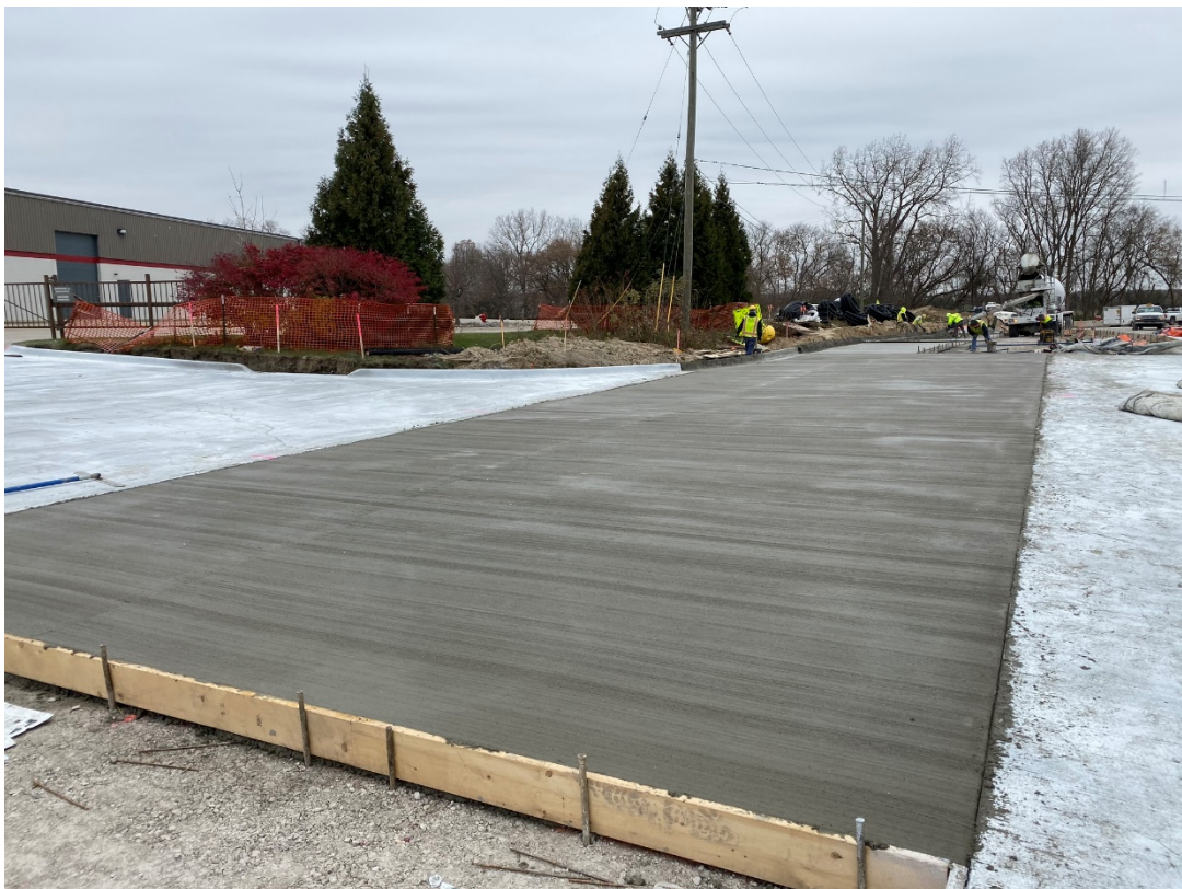
Pouring the southbound lanes of Crescent Boulevard and driveway for General Filters.
