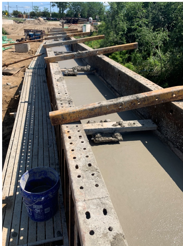
Wall forms and poured concrete for Crescent Boulevard, SW corner of river.
