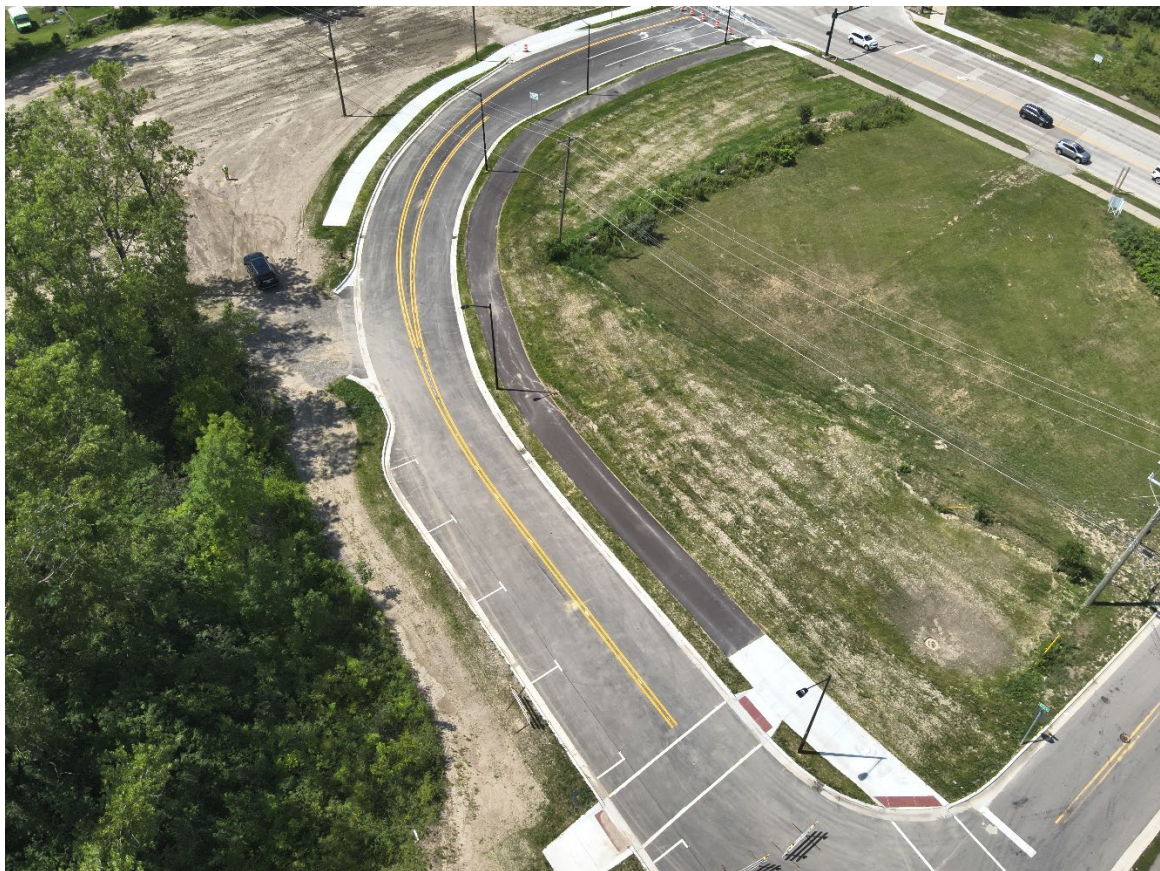
After – Overall aerial photo looking northwest
