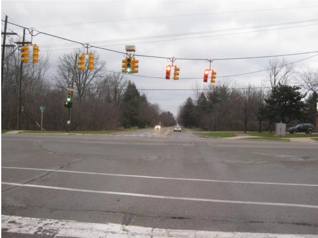
11 Mile Road Facing East
