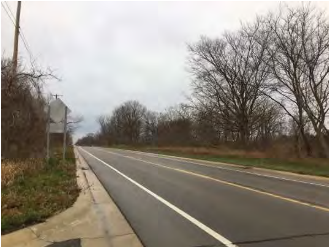
LOOKING EAST ALONG W. EIGHT MILE ROAD
