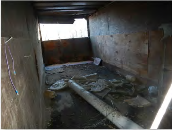
On site tool trailer with debris.
