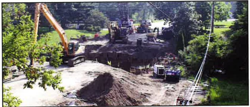
The view of the Wise Road culvert project from the work zone camera.
