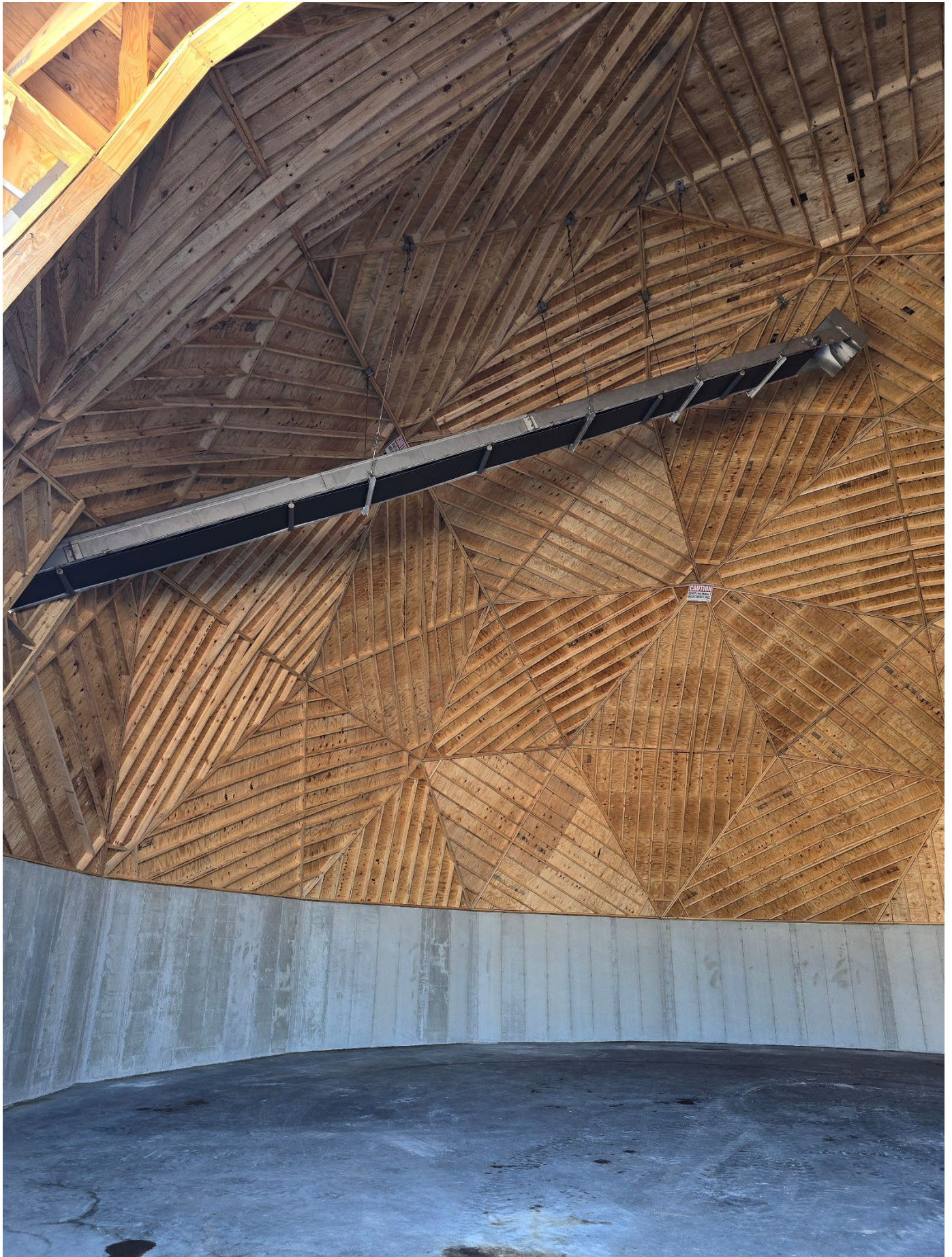
New interior dome shell, 10-foot high concrete walls, and conveyor system (7-18-25)
