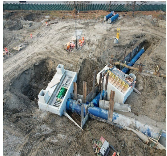
Figure 2: 48-inch WM and GV Installation
