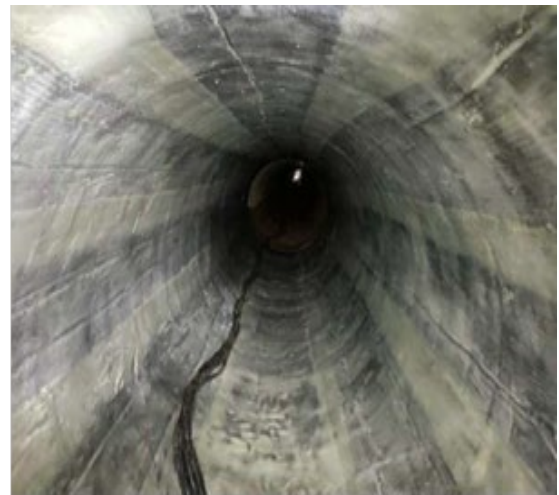
Figure 6: CFRP Partial Install
