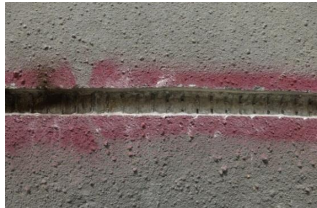
Figure 2: Cutting of Prestressing Wires
