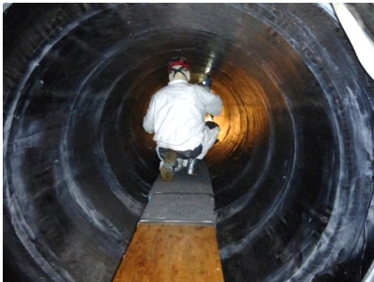
Figure 1: Installation of V-Wrap FRP Liner
