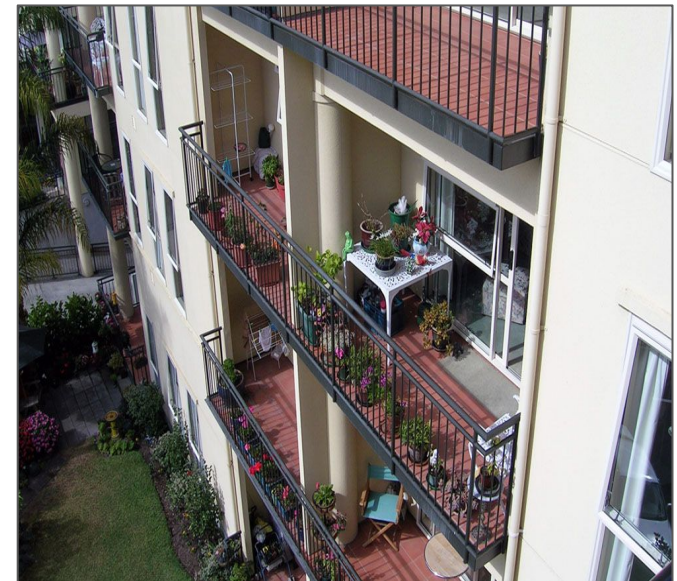
Dedicated outdoor space for every unit
