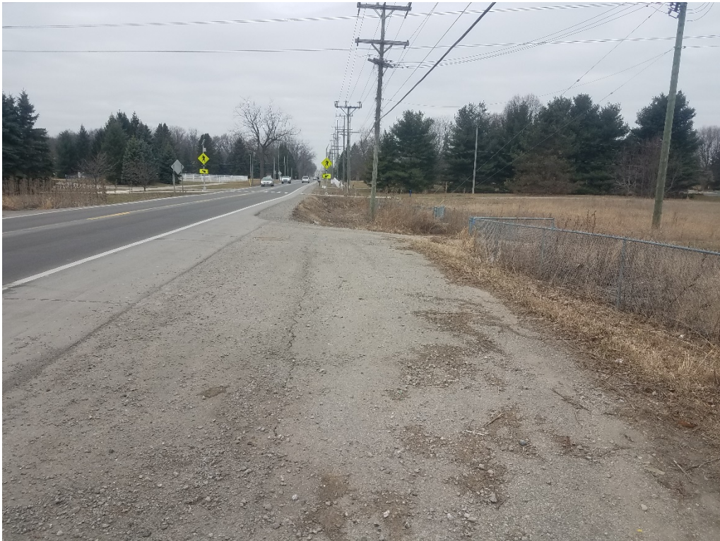
Before – At the ITC Corridor, looking west
