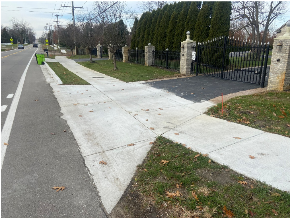
After – East of the ITC Corridor, looking west
