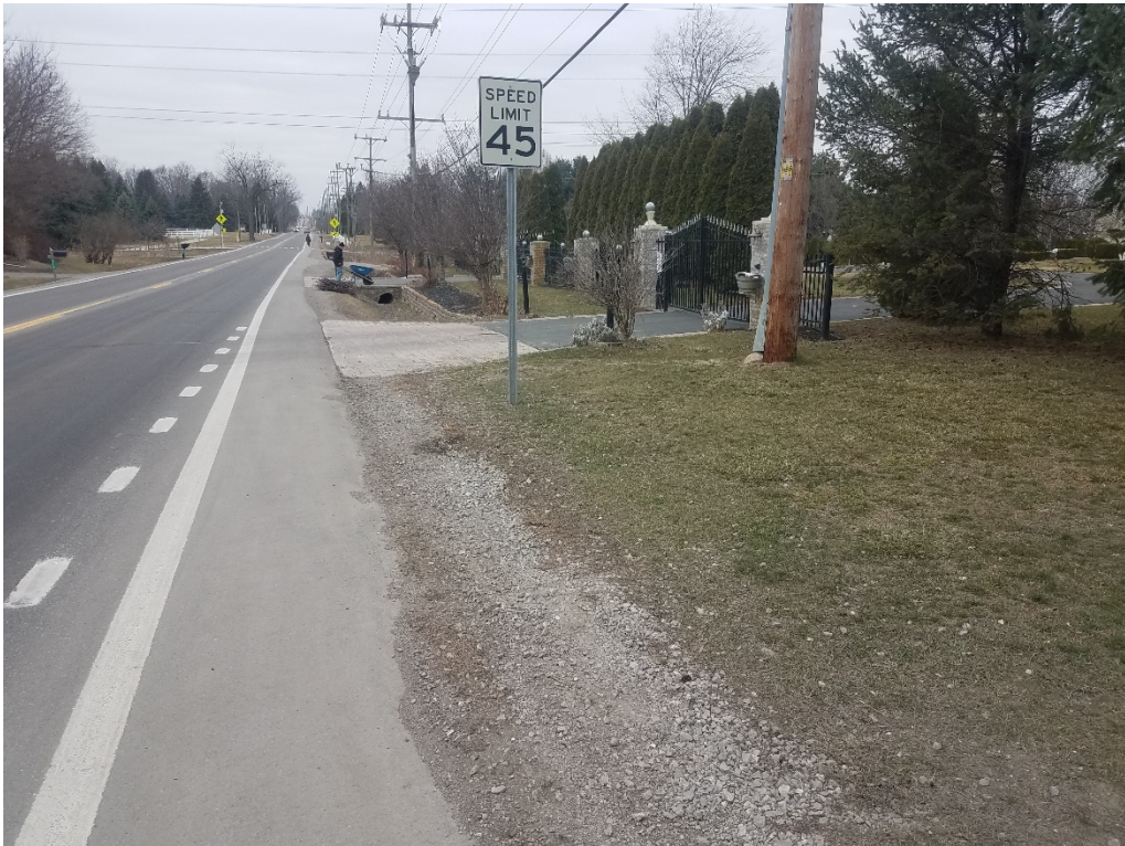
Before – East of the ITC Corridor, looking west
