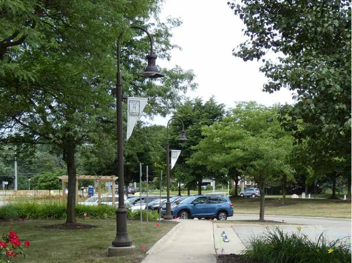
Existing pedestrian walkway lights
