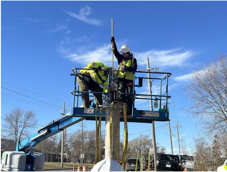
Figure 5: PipeDiver Pressurized Insertion Stack
