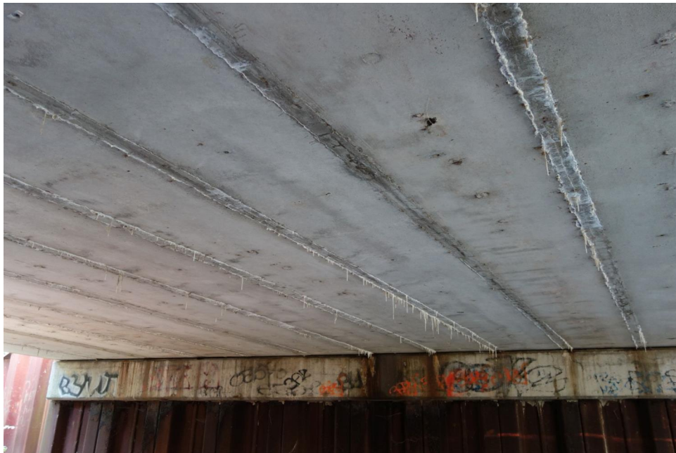
Typical Deck Underside
