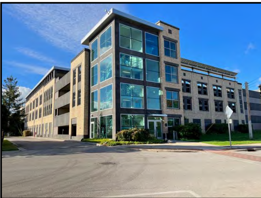
Figure E26: Parking structure in Traverse City
