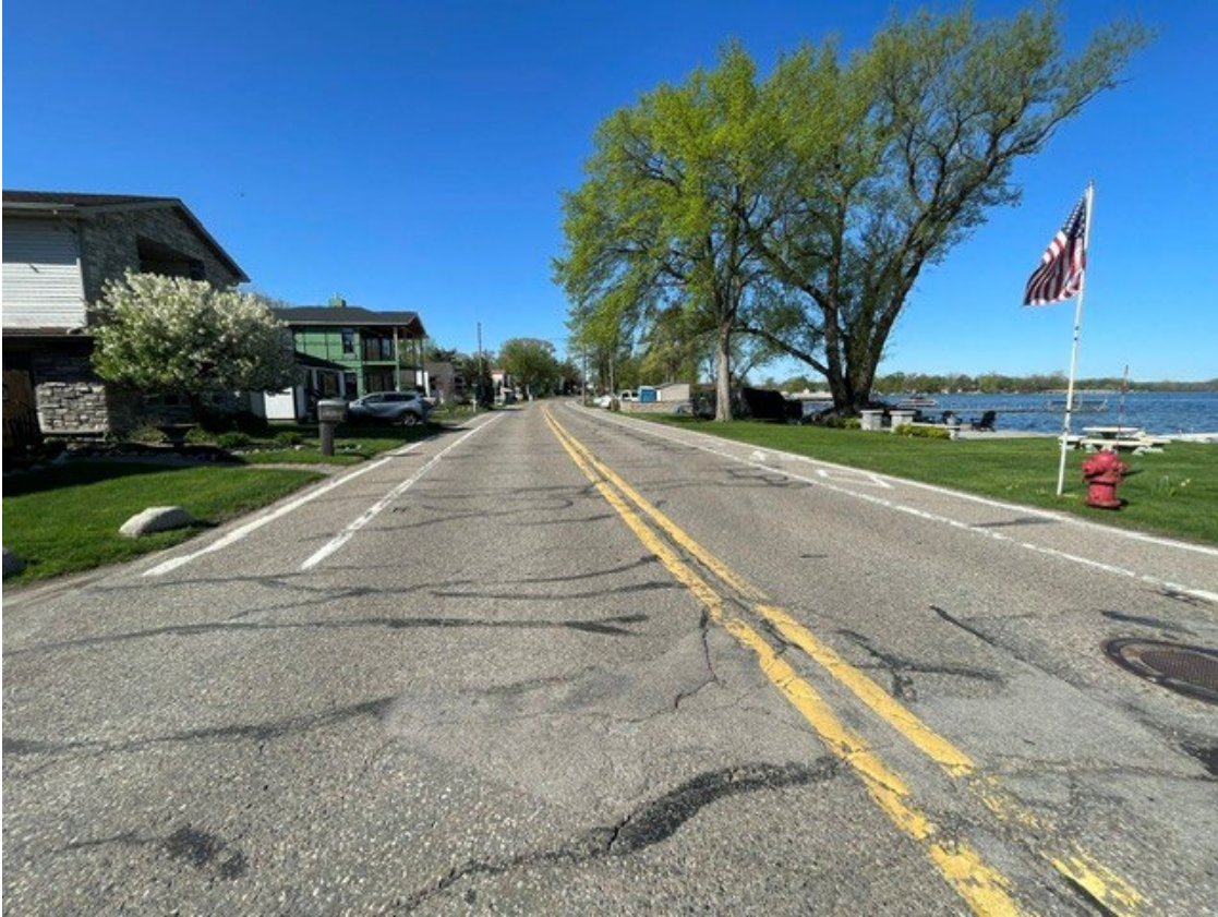
Before: East Lake Drive looking west from Lashbrook Street
