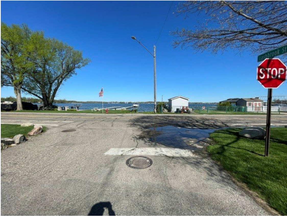
Before: Monticello Street at East Lake Drive
