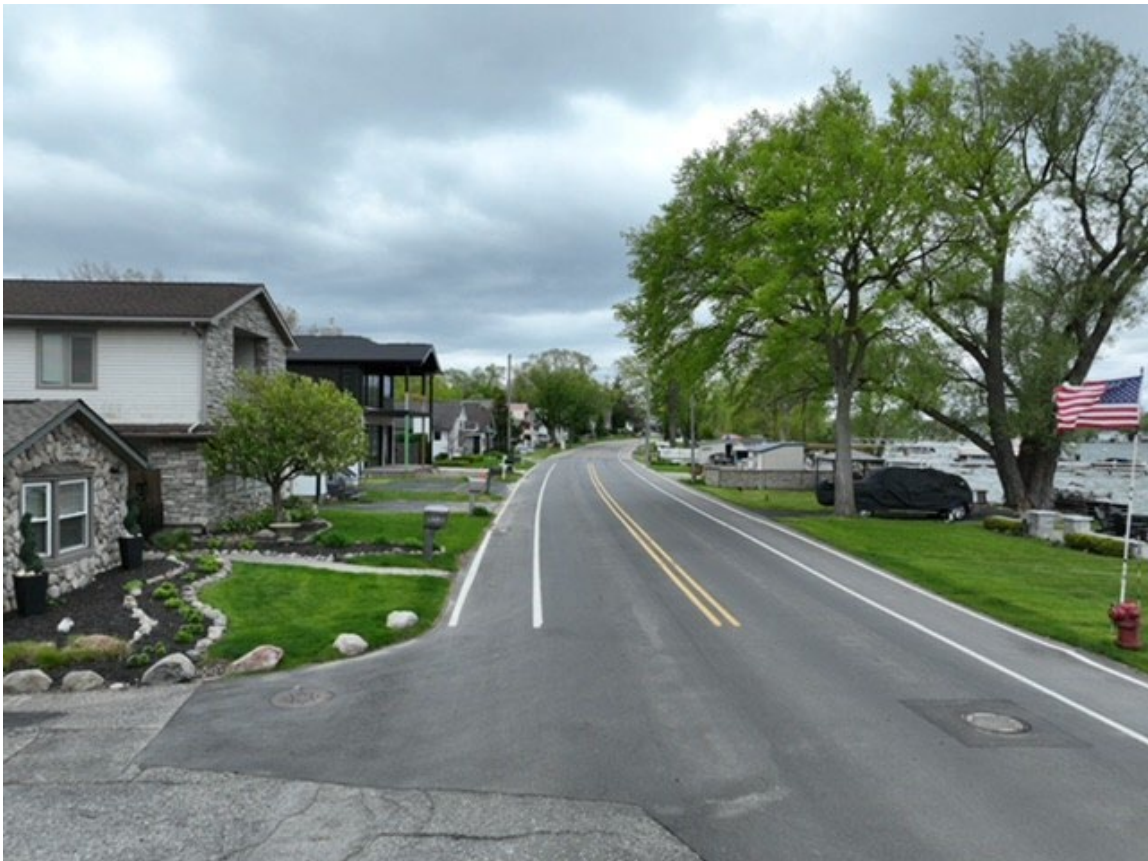
After: East Lake Drive (drone picture) looking west at ground level from Lashbrook Street
