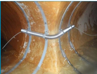
Bend protection in-pipe
