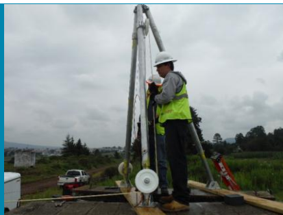
Feeding cable into the pipeline
