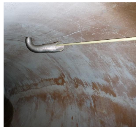
Cable protection into pipe
