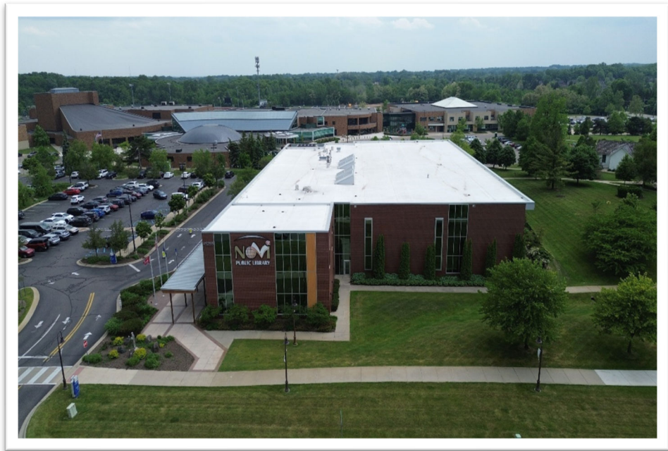
Photograph 2: Typical view of building exterior elevation
