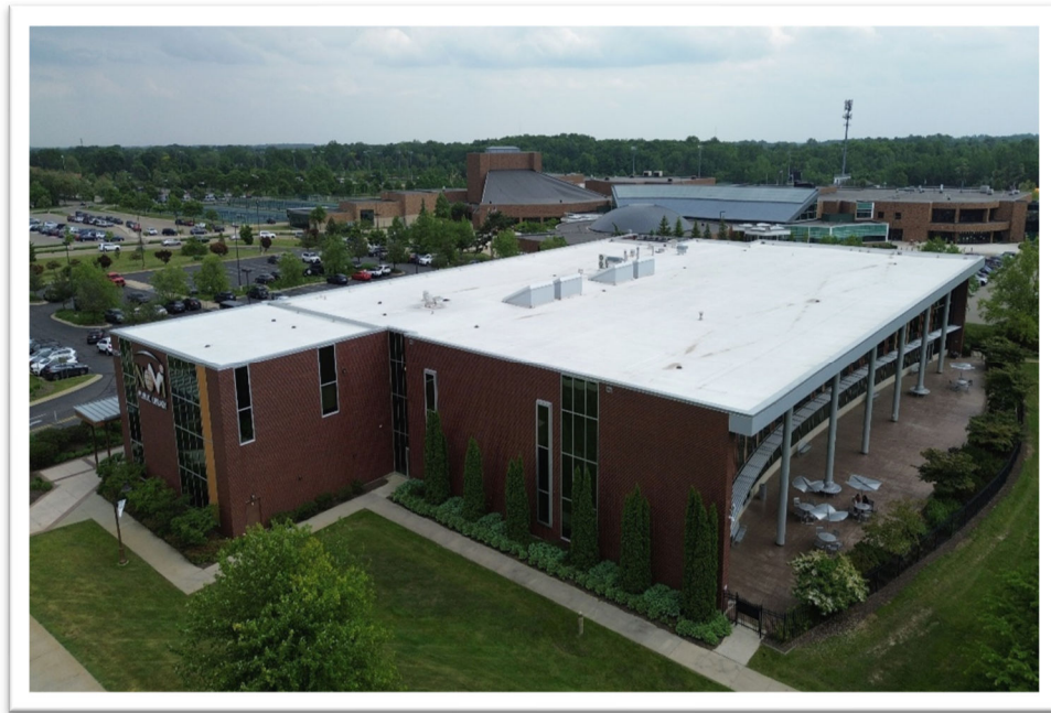
Photograph 3: Typical view of building exterior elevation
