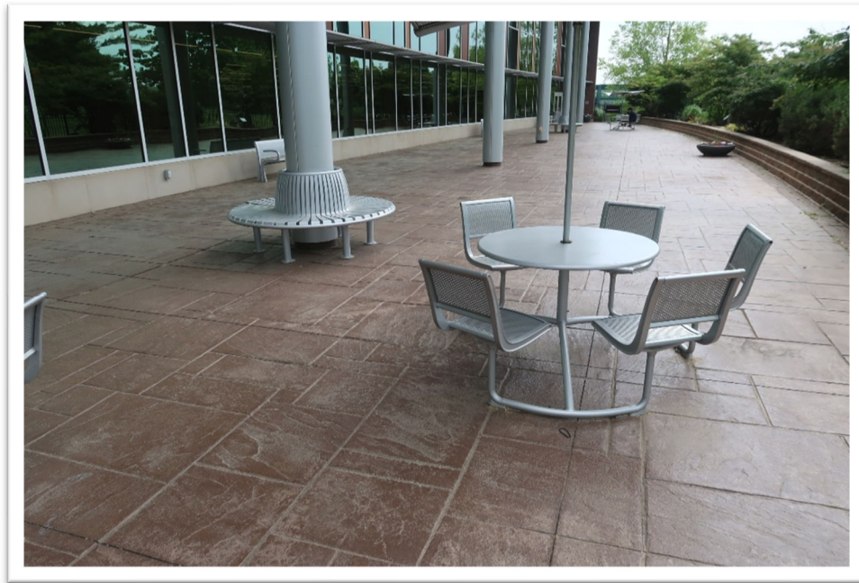
Photograph 27: Typical view of stamped concrete patio area
