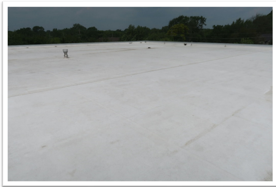
Photograph 5: Typical view of TPO membrane roof cover
