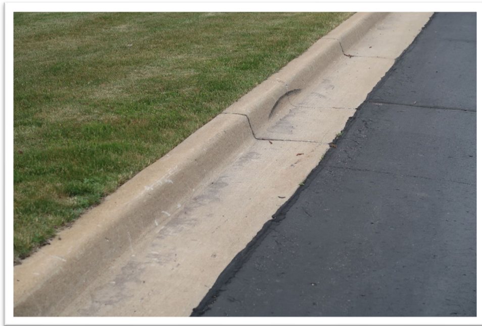
Photograph 29: Typical view of concrete curb
