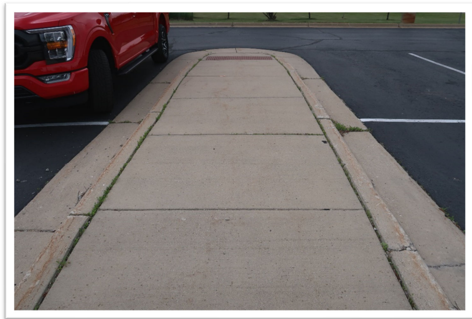
Photograph 26: Typical view of concrete sidewalk
