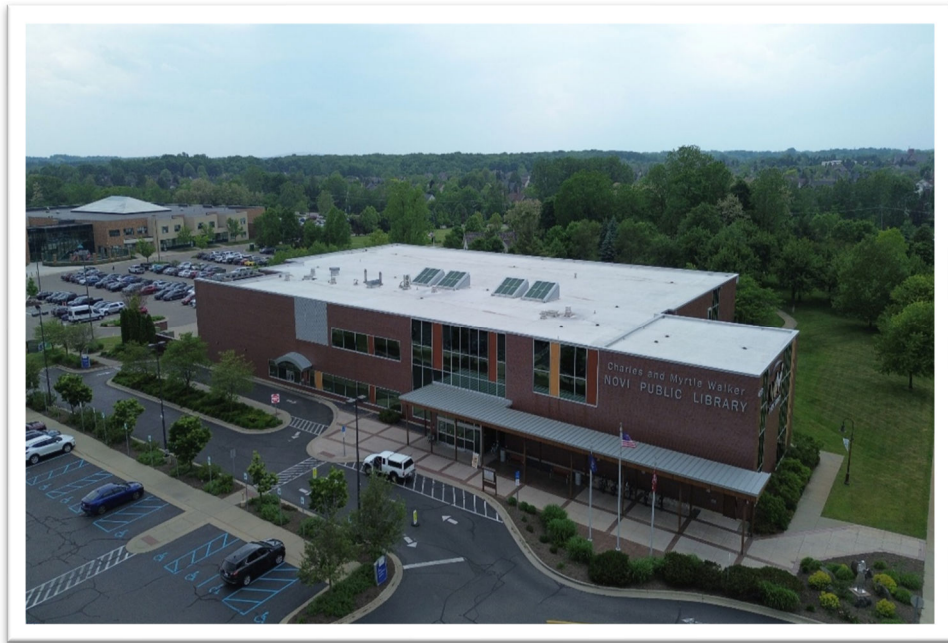
Photograph 1: Typical view of building exterior elevation
