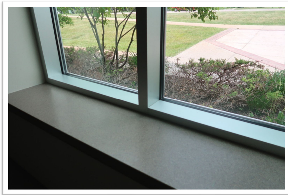
Photograph 9: Typical view of window
