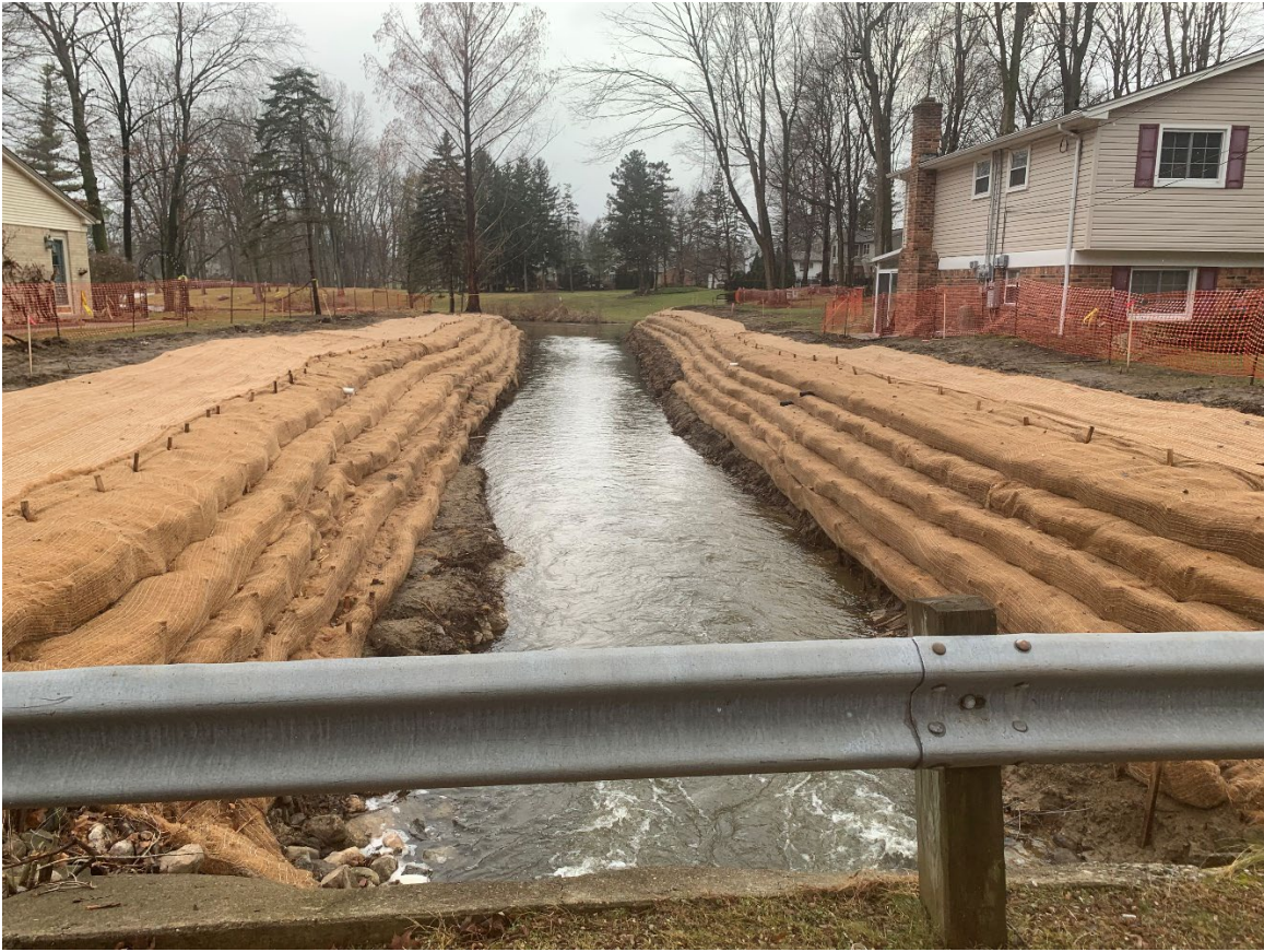
Looking south at Middle Rouge River from Chattman Drive during streambank stabilization
