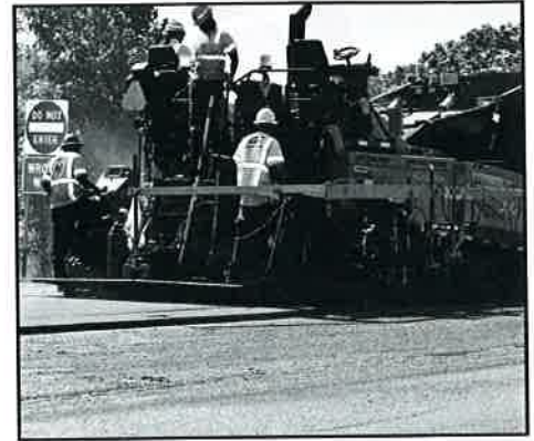
A paving contractor completing an RCOC Preservation Overlay.
