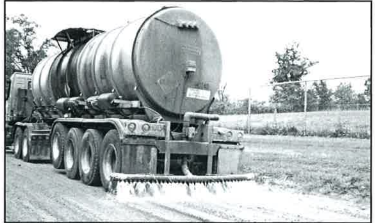
An RCOC tanker applying brine for dust control on a gravel road. New EGLE rules would restrict dust-control.
