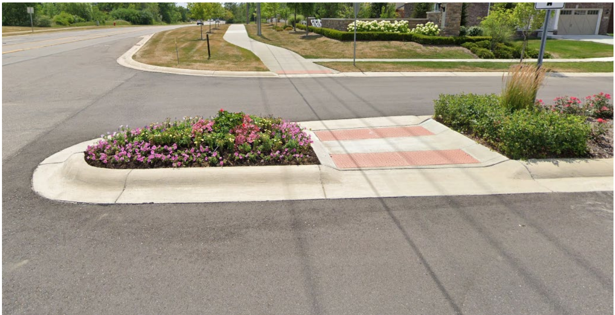
Pic 3: Front Island Flower Bed – with sprinkler set up
