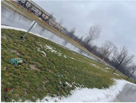
Pic 4 : After- construction work. Sod Along the Wixom Road
