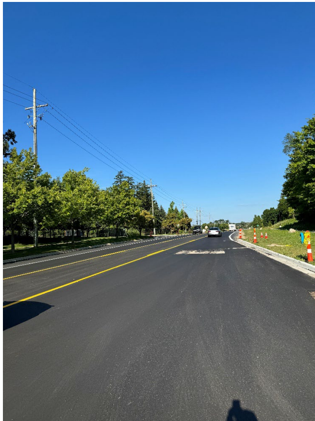
After - Completion of 13 Mile Road paving at Fox Run Village
