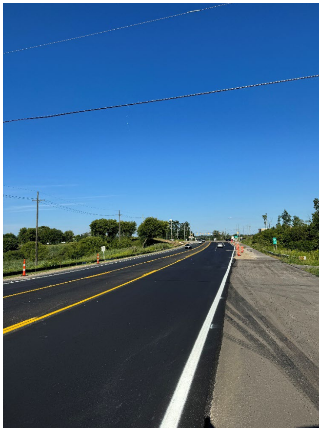
After – Looking towards the intersection of 13 Mile Road and M-5
