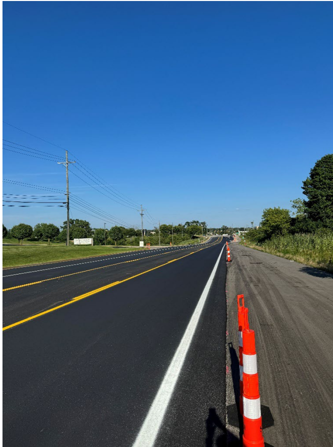
After - Completion of 13 Mile Road paving at Brightmoor Tabernacle Church entrance
