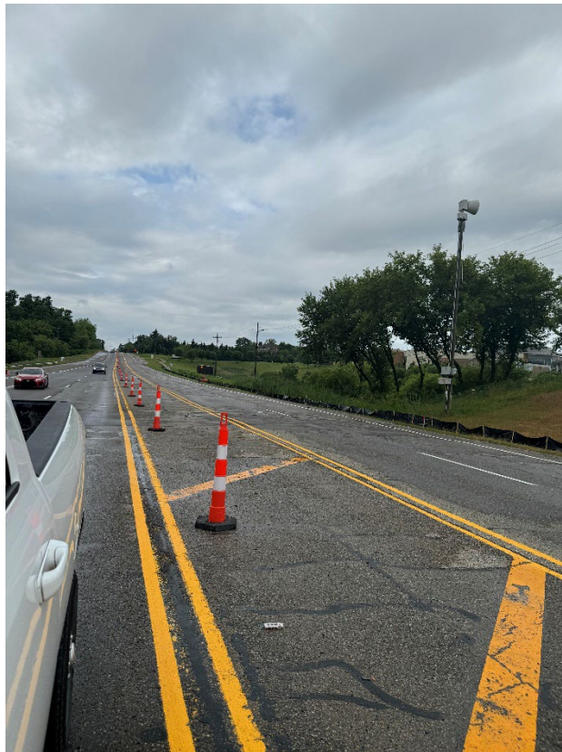
Before – 13 Mile Road looking east from Meadowbrook Road
