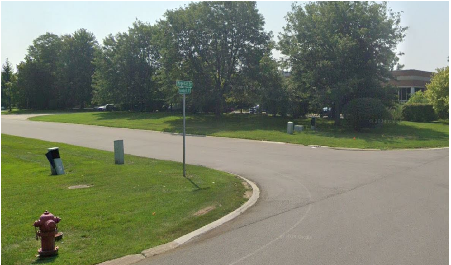
After – Completion of the intersection of Magellan and Humboldt Drives.
