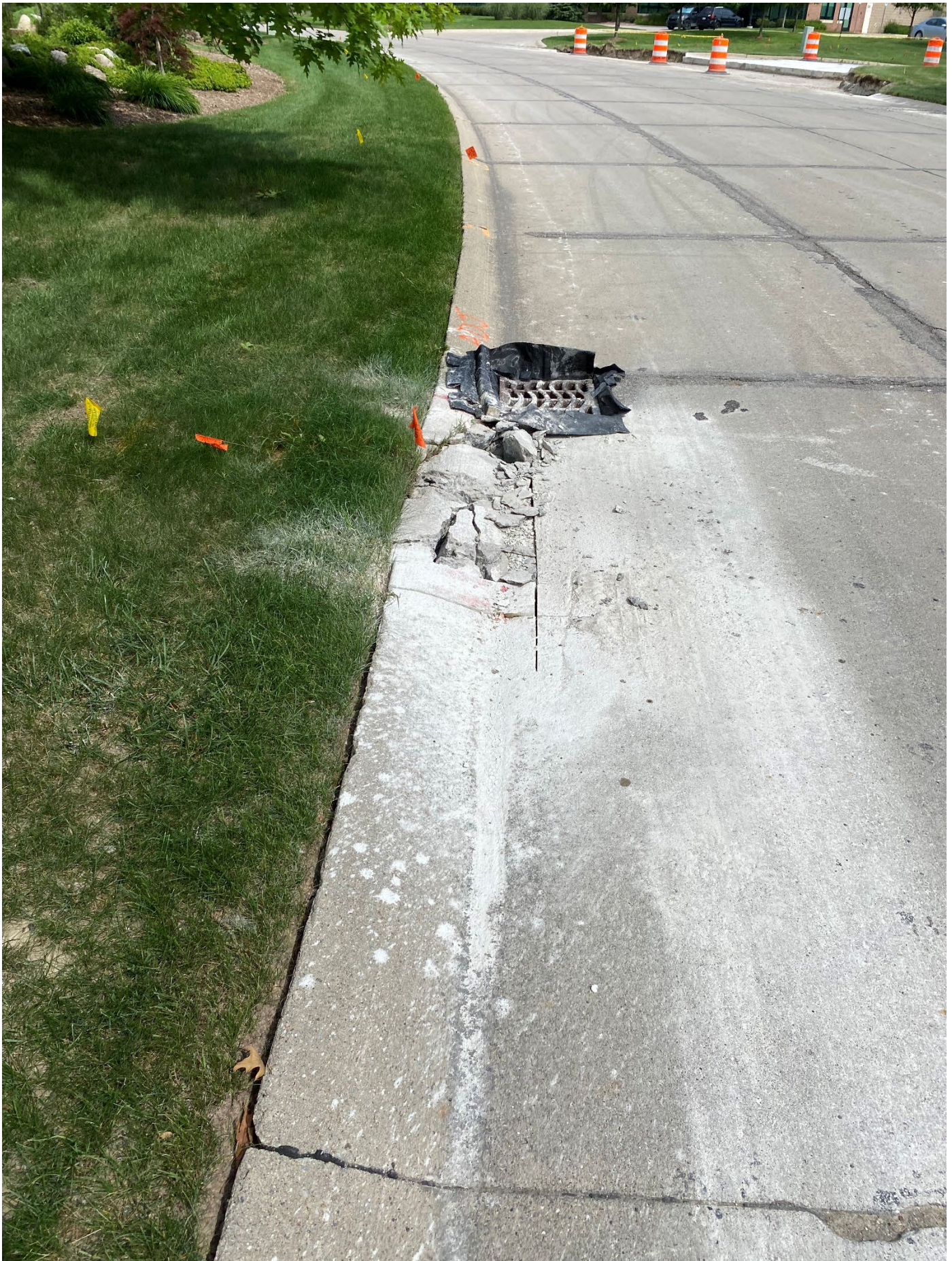
During – Saw cutting and preparation work on existing concrete in the Beck West Corporate Park
