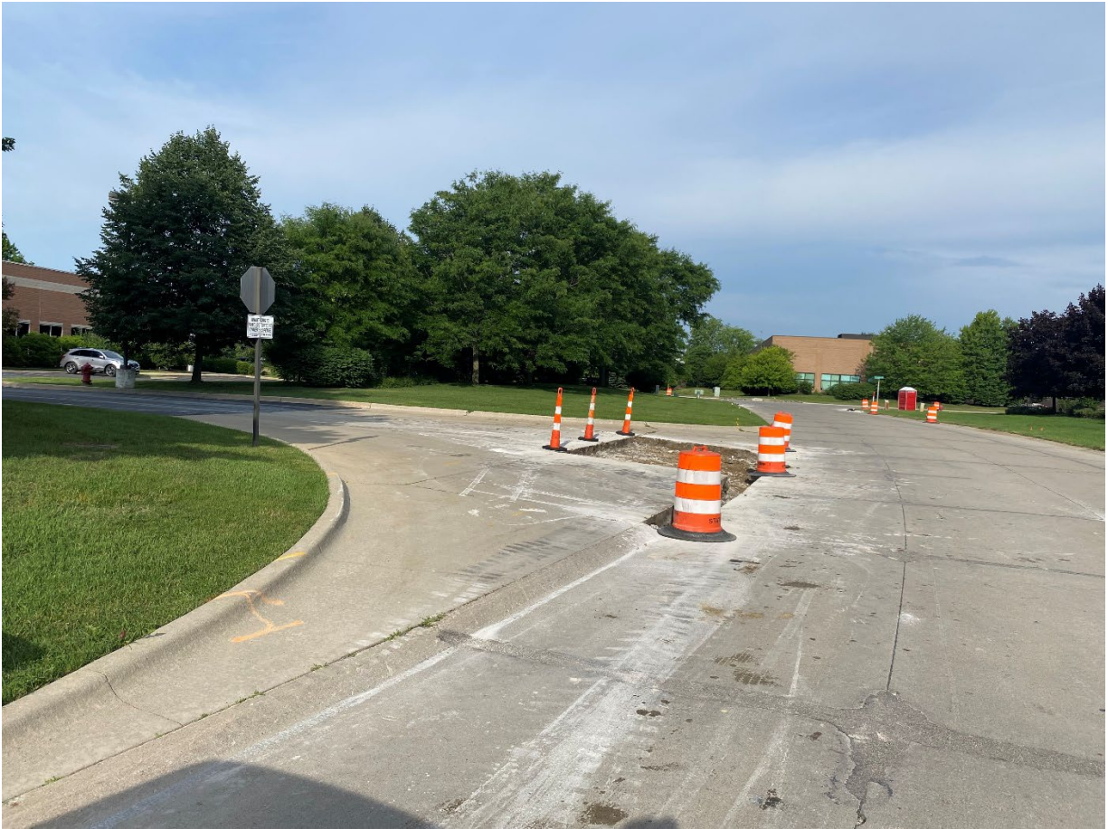
During – Existing concrete pavement removals and condition on Hudson Drive
