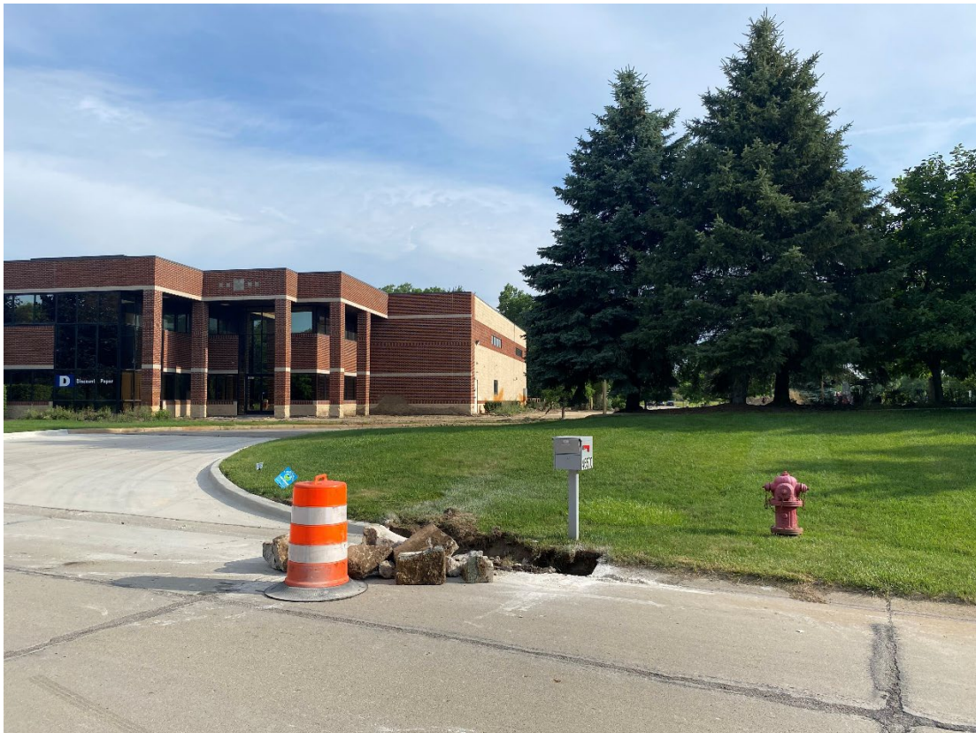
During – Existing concrete pavement removals and condition on Peary Court
