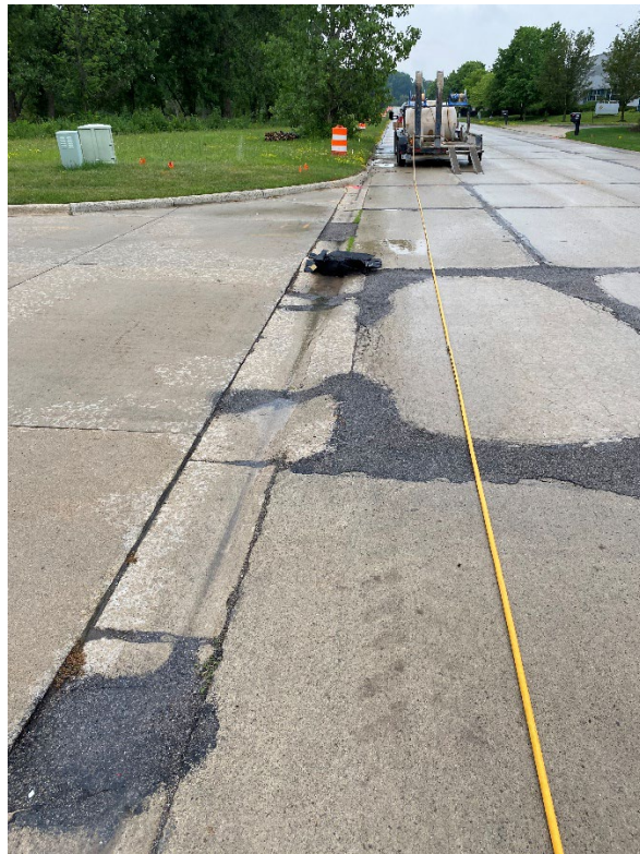
Before – Drive and curb line pavement on Magellan
