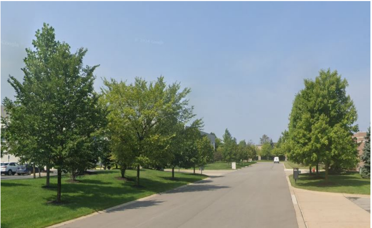
After – Completion of Peary Court in the Beck North Corporate Park
