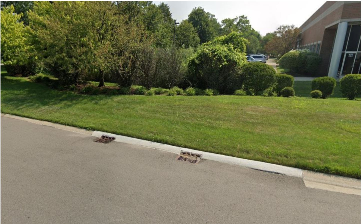
After – Drive and curb pavement completed on Magellan Drive
