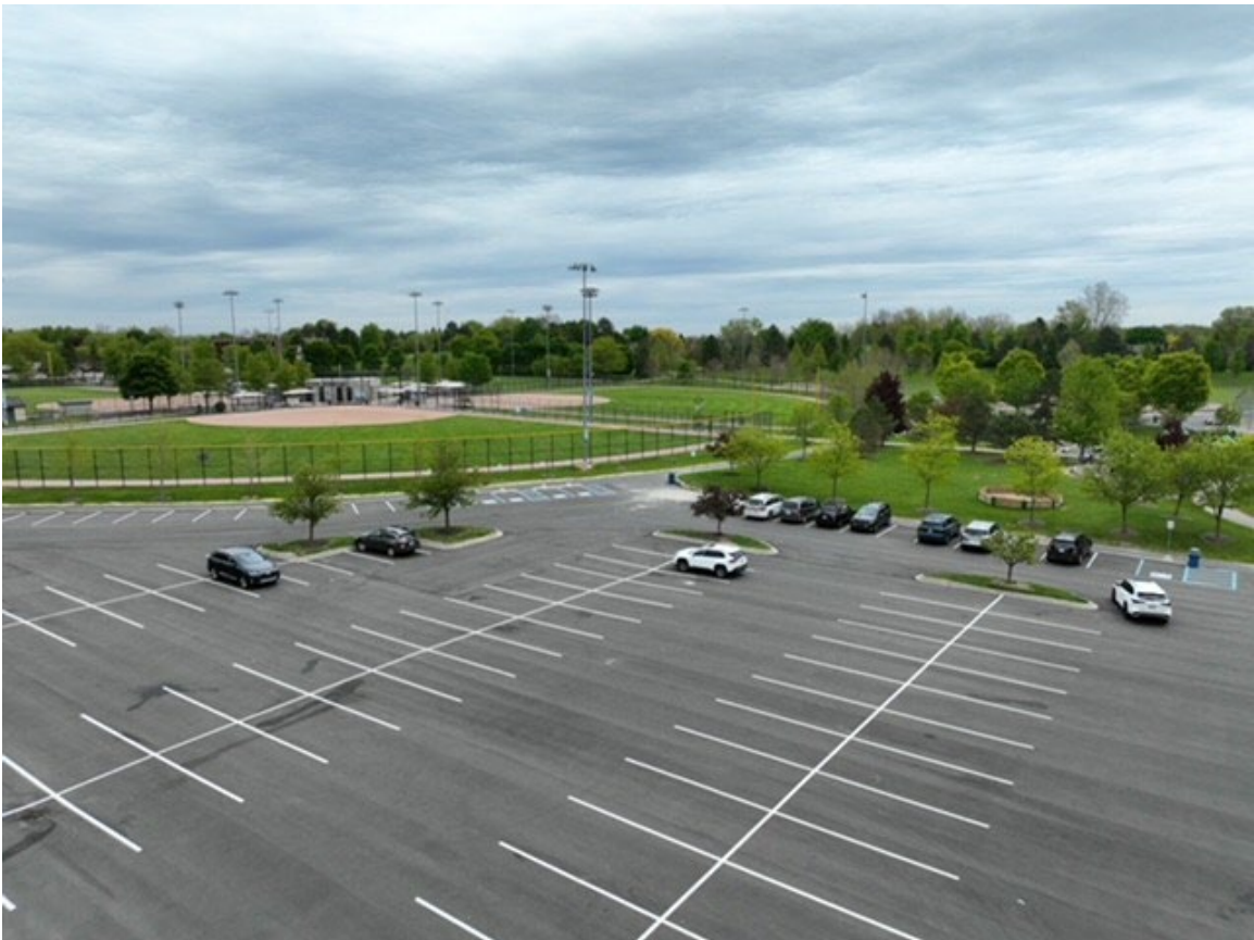
After: Drone image of parking lot looking northeast
