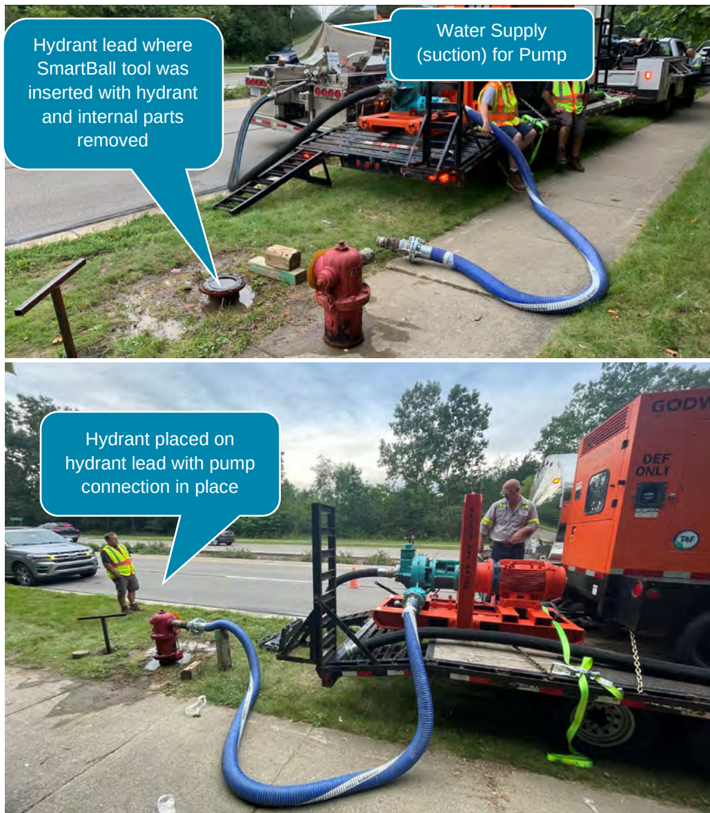
Figure 2.3: View of SmartBall Insertion Location, Pump used to push SmartBall Tool into the Main
