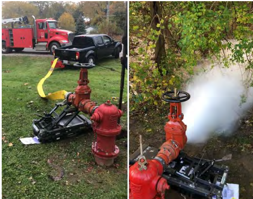
Figure 2.3: Fire Hydrant Configuration
