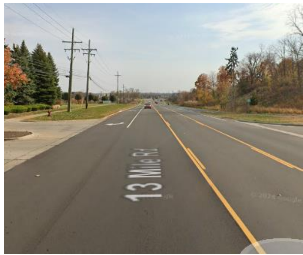
13 Mile Rd - After
