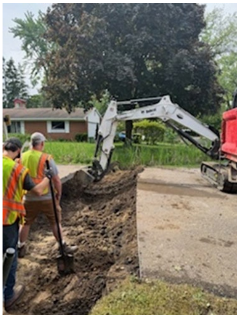
Removing and replacing culverts between ditches
