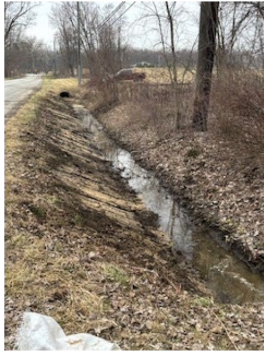
Cleaning a ditch full of sediment
