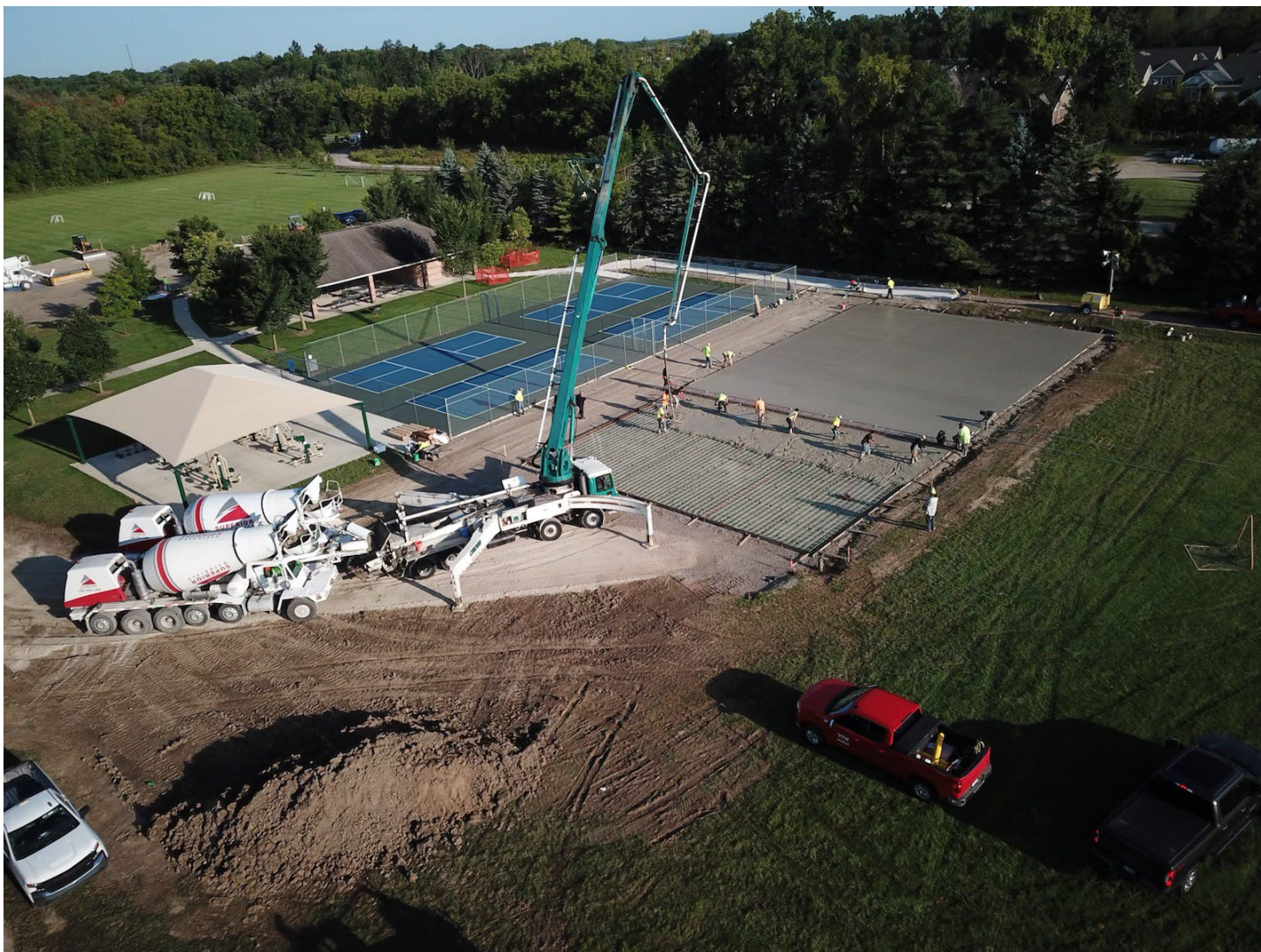
During – Pumping concrete for new courts
