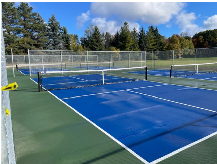
After – New courts complete
