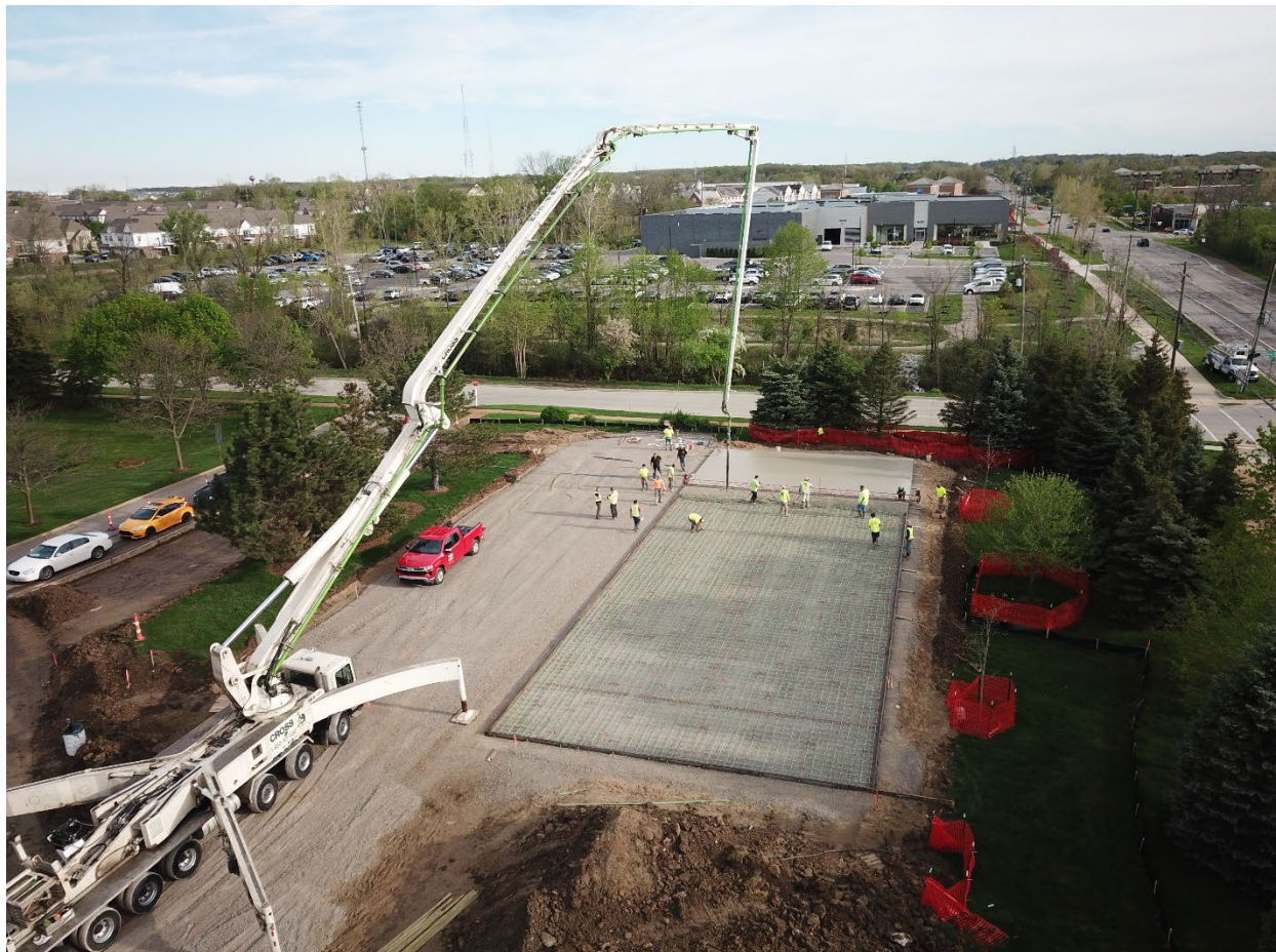
During – Pumping concrete for new courts
