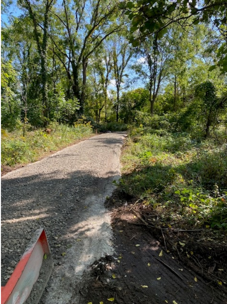
Pic 3 Wooded pathway construction with gravel – not yet tamped down
