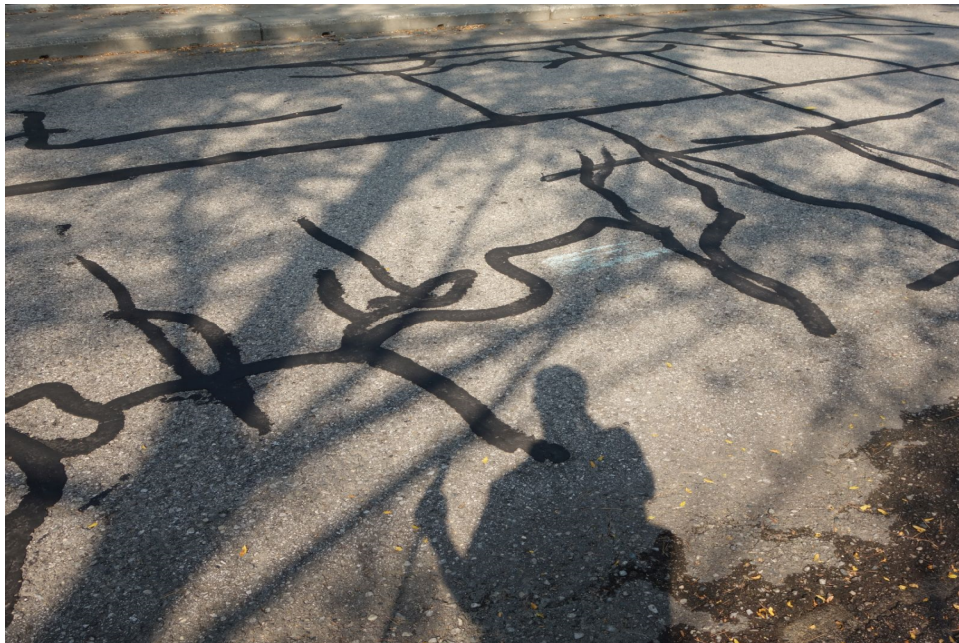
Typical Deck Surface
