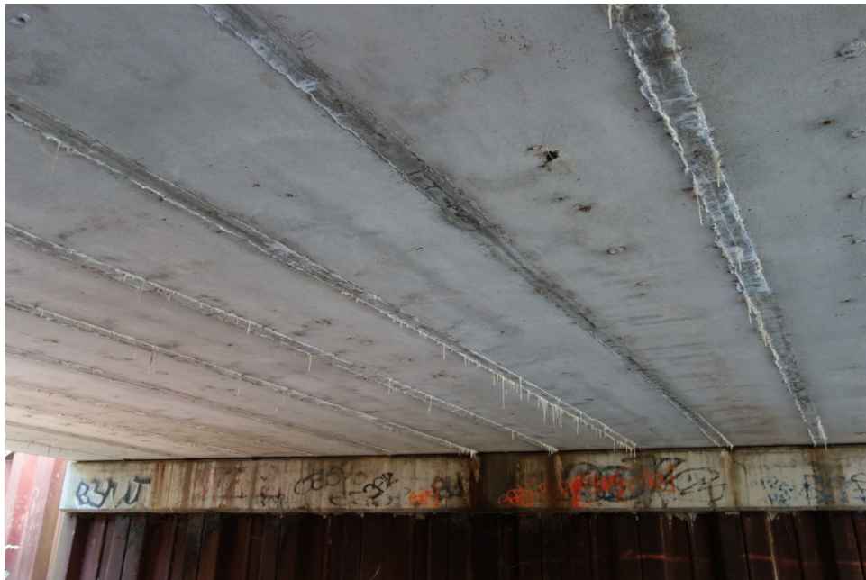
Typical Deck Underside
