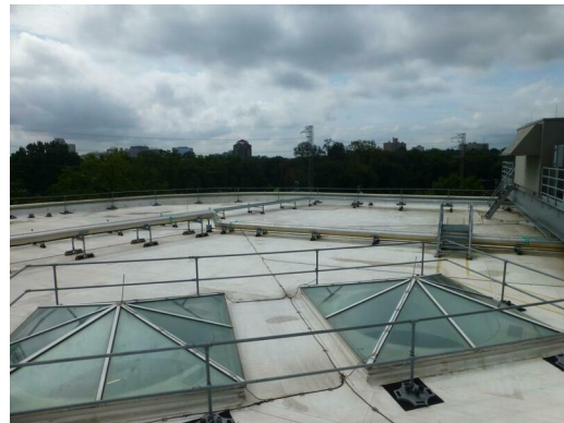
Rooftop at Bldg 1
