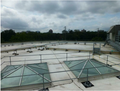
Rooftop at Bldg XXXX
