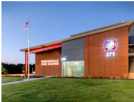
DUNCANVILLE, TX FIRE STATION NO. 1
