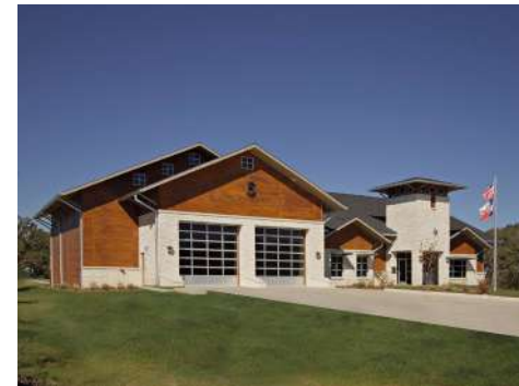
COLLEGE STATION, TX FIRE STATION NO. 5
