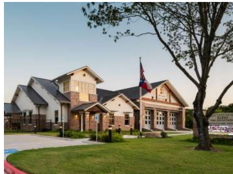
KLEIN, TX FIRE STATION NO. 3
