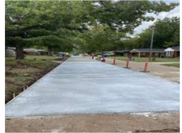
Caddell Lane (Urban Concrete)
