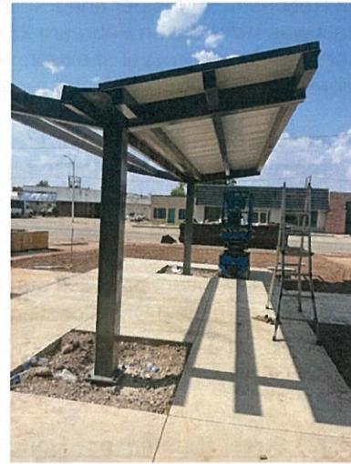
Seating structure assembly
