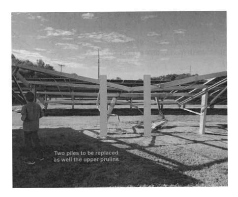
Acquire replacement OMCO racking of same type, reinstall new piles, new tables/purlins, and install 14 new panels, and redo stringing into inverter
