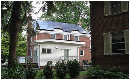
Not recommended - solar roof panels have been installed at the rear, but because the house is situated on a corner, they are highly visible and negatively impact the character of the historic property. (Source: NPS)
