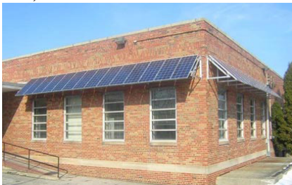
Solar panels, which also serve as awnings, were installed in secondary locations on the side and rear of this historic post office and cannot be seen from the front of the building. (Source: NPS)
