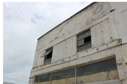
Broken glass should be replaced, and features such as canopies should be replaced where they existed originally.
