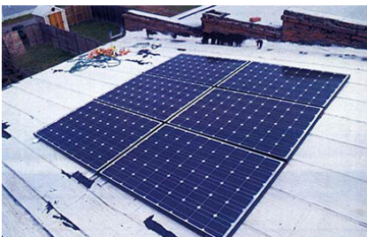
Solar panels were installed appropriately on the rear portion of the roof on this historic house that are not visible from the primary elevation. (Source: NPS)
