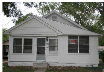
Wood windows should be repaired and not replaced with aluminum frame windows.
