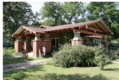
Brick has an inherent natural color and should not be painted or sealed.
