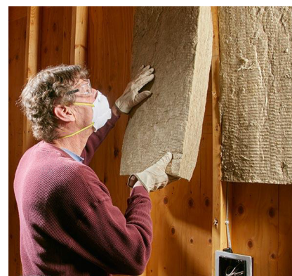
Mineral wool is also an appropriate insulation material.
