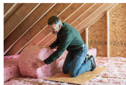
Fiberglass batt is an appropriate insulation material.
