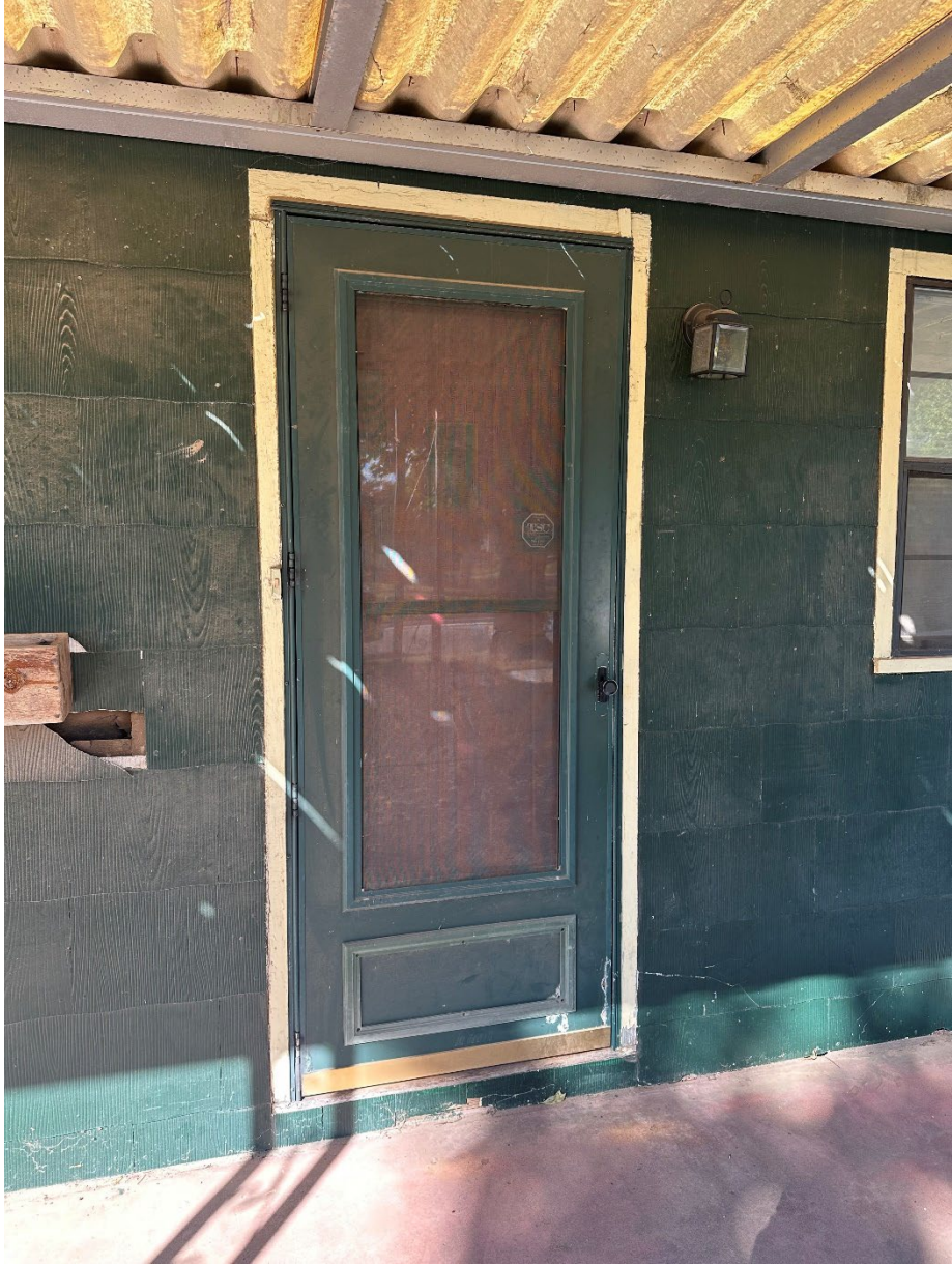
Storm door to be replaced with Aluminum full view storm door.
