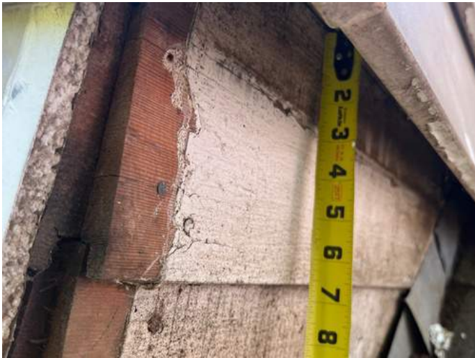
Underlying shiplap siding (will leave and install over)
