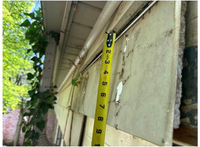
Existing metal siding dimensions
