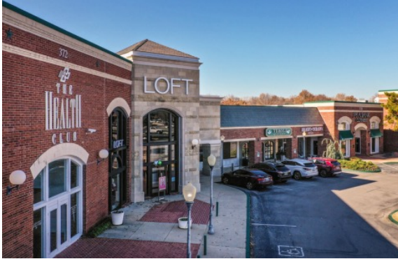
Brookhaven Village Building E
