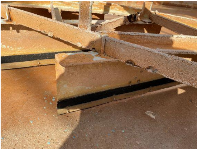
Turnbuckles severely corroded
