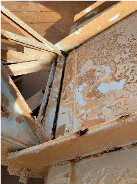
Steel pitting in scraper truss
