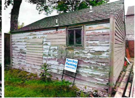
REAR (EAST) – ACCESSORY STRUCTURE
