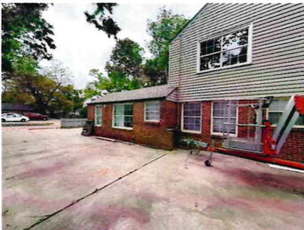
SOUTH – PRIMARY STRUCTURE
