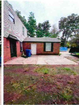
NORTH – PRIMARY STRUCTURE
