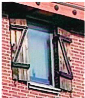
New wood stained shutters at windows
