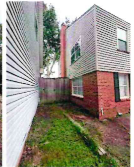
NORTHWEST – PRIMARY STRUCTURE
