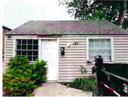
FRONT (WEST) – ACCESSORY STRUCTURE
