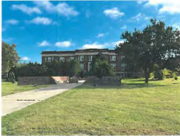
Old Administration Building Preservation
