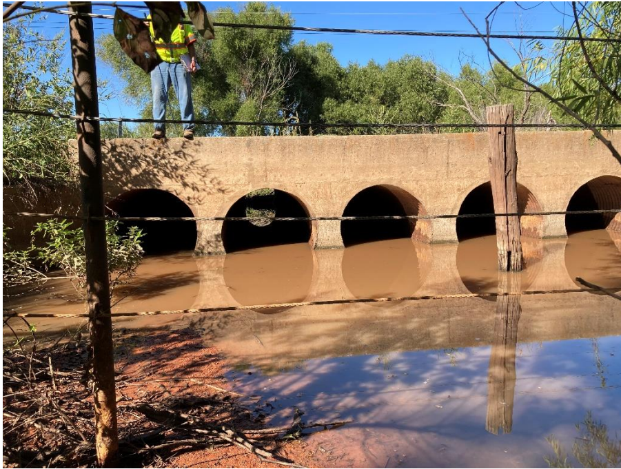
Elevation view, looking north
