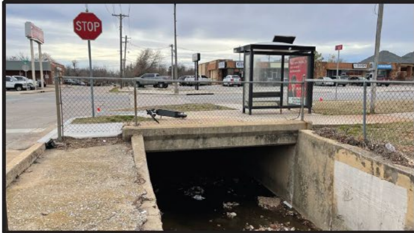
Figure 1. Culvert over Imhoff Creek at location I1.
